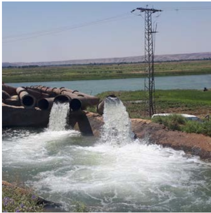
Pipes fill an irrigation canal from the Euphrates River. Photo credit: USAID Syria Essential Services II program
