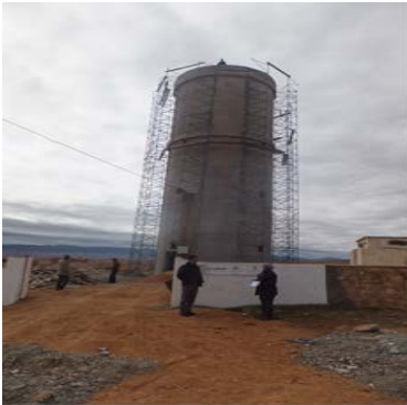
Aghbalou Water Tower in construction (Photo: ADPE)
