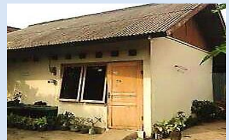
Transitional shelter provided in 2006 after the magnitude 6.3 earthquake in Java, Indonesia, upgraded to permanence. See summary of SSWG post-project “ten years on” review. Photo courtesy of InterAction
