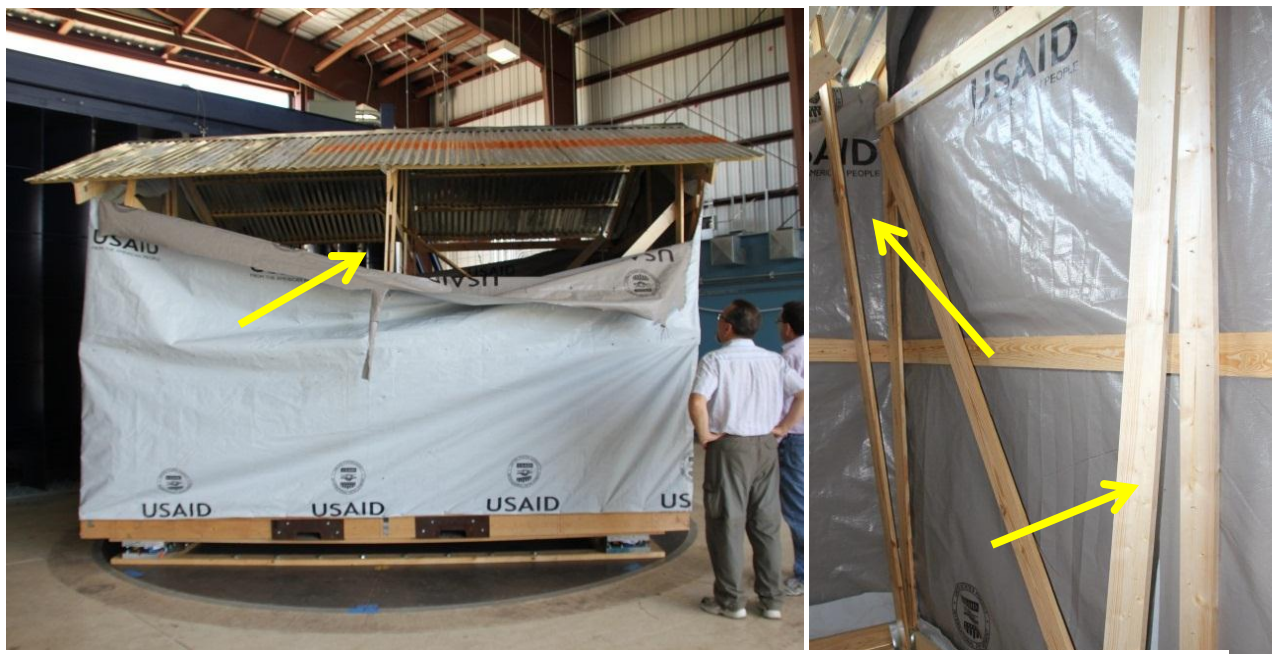
Figure 24 - Nail pull-out failure on shelter framing at 75 mph
