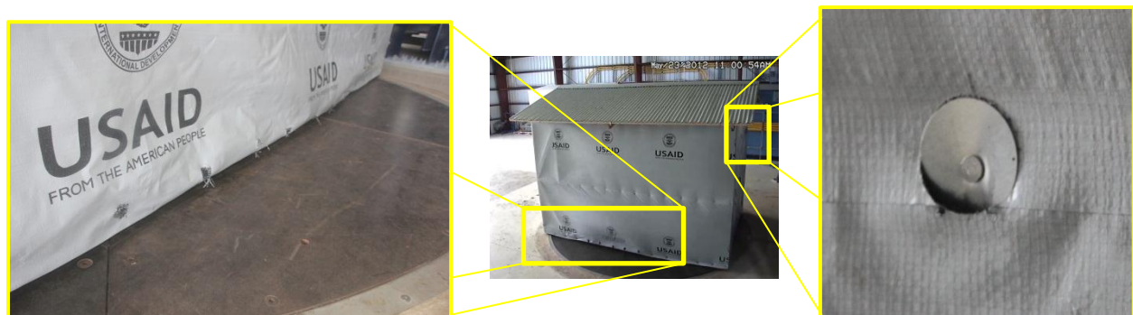
Figure 7 - Plastic puncture by tin cap discs
