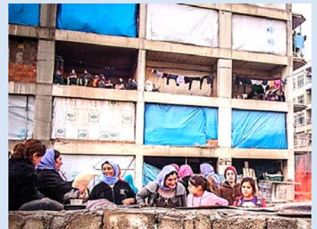
USAID/OFDA provided closing-off kits to help turn multi-story, unfinished commercial buildings in northern Iraq into adequate emergency shelter for displaced populations. Photo by USAID/OFDA
