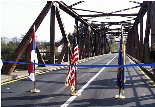
Following the 1992-1995 war in BiH, USAID assistance focused on reconstruction of infrastructure, including major bridges.
