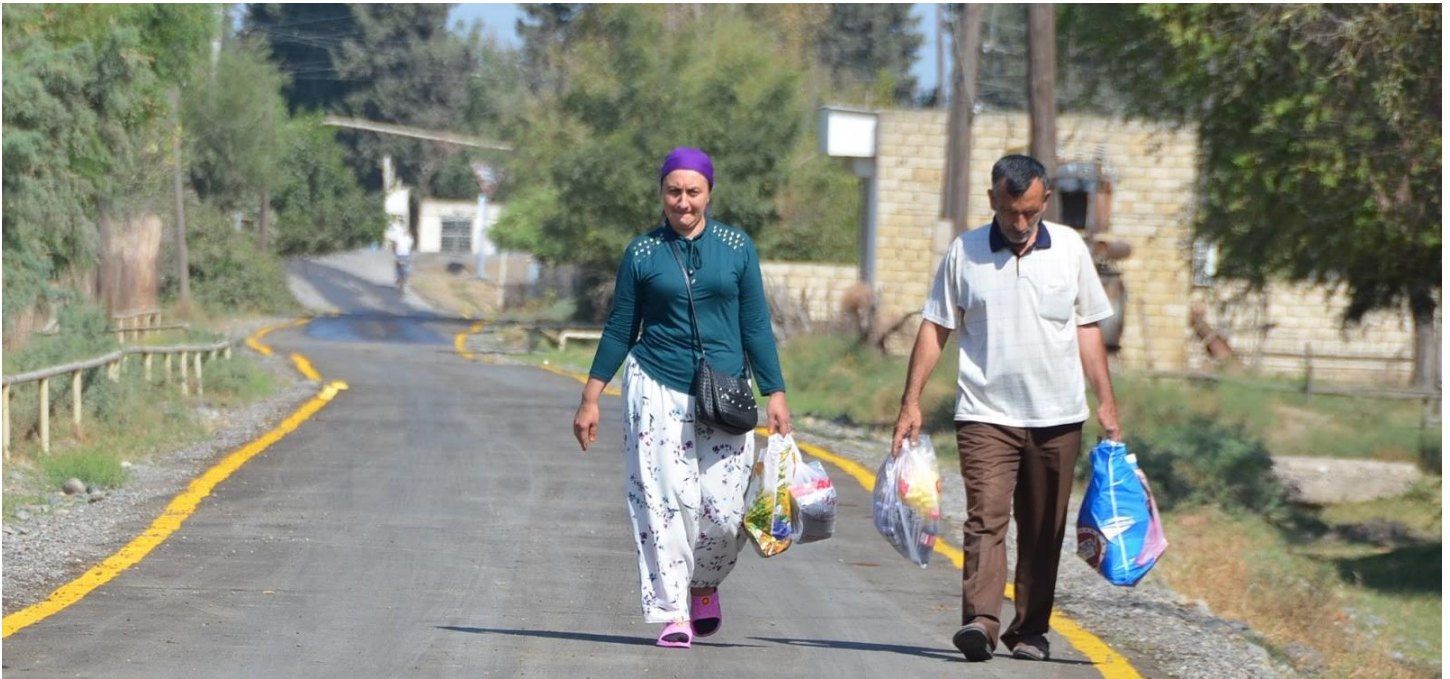
Residents of the Varkhan community in central Saatli district using the new road renovated with support from USAID and the Azerbaijani government through SEDA. Photo: Vugar Naghiyev/USAID Azerbaijan
