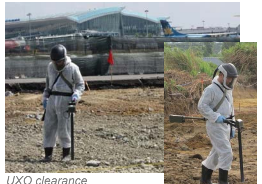
UXO clearance (Photos: CDM Smith)
