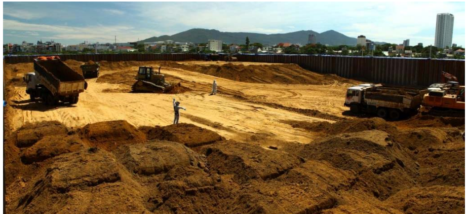
Placing contaminated soil and sediment in containment structure (Photo: CDM Smith)
