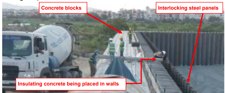
Pouring insulating concrete into the containment structure walls (Photo: CDM Smith)
