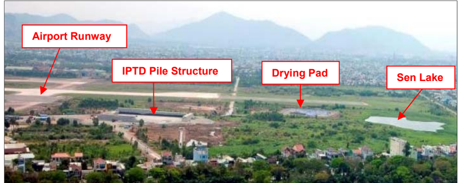
Panoramic view of the project site, looking west (Photo: David Liu, Tetra Tech)
