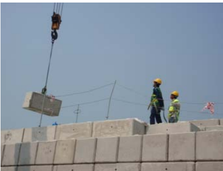
Fall protection equipment (Photo: CDM Smith)
