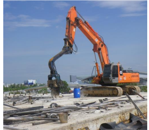
Removing thermal treatment system equipment from the structure (Photo: CDM Smith)
