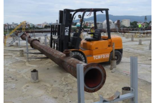
Removing vapor manifold from Phase 1 treatment structure (Photo: CDM Smith)
