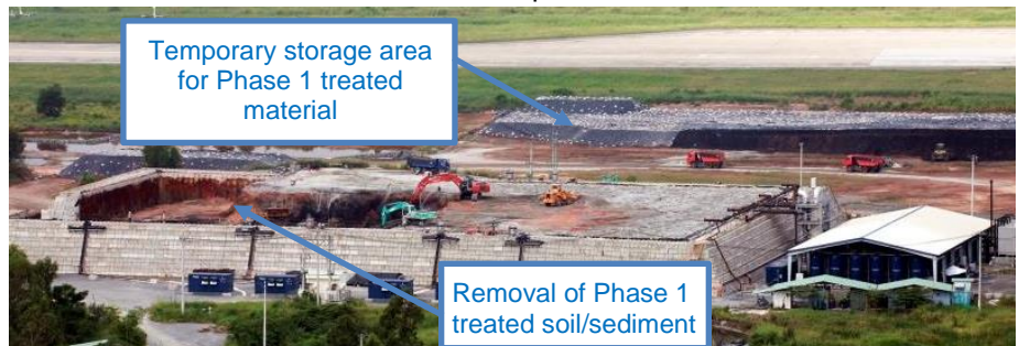
Removal and temporary storage of Phase 1 treated material (Photo: Tetra Tech)
