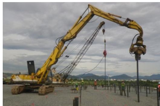
Installing heaters into pile structure (Photo: CDM Smith)
