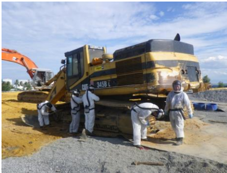
Decontaminating equipment before leaving project area (Photo: CDM Smith)
