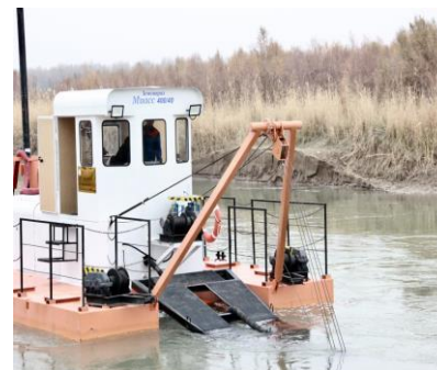
The dredger, funded by USAID, will help prevent flooding in Mary, Turkmenistan.
