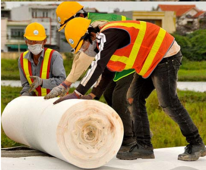
Workers complete site preparation at Danang Airport.
