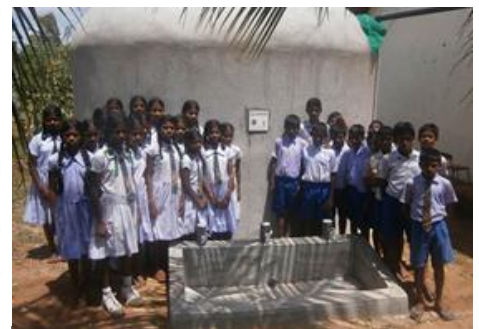
U.S.-supported rainwater harvesting systems help rural, drought-prone schools access water in Sri Lanka. Photo credit: Lanka Rainwater Harvesting Forum
