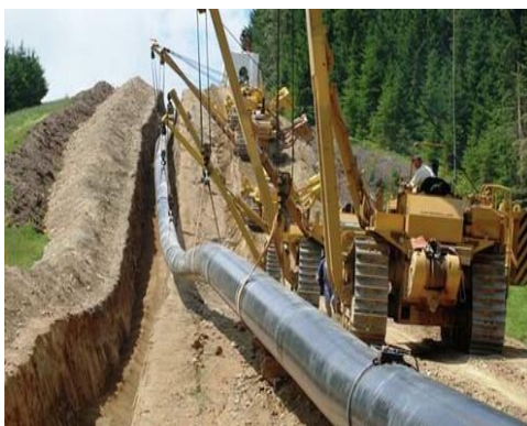
West African Gas Pipeline construction
