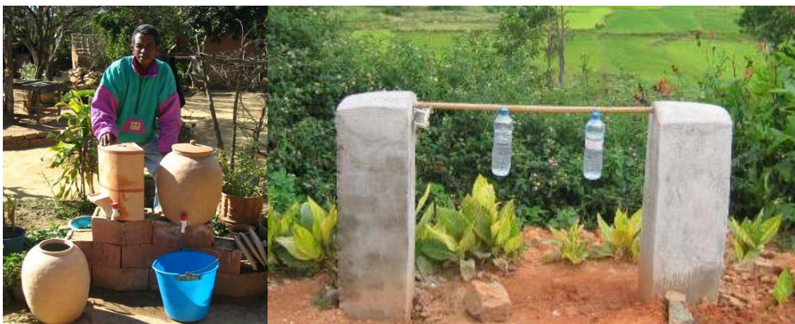
Examples of simple handwash stations: above: earthenware pots with spigots; below: suspended PET bottles. These designs do not require plumbing, but do require effective management to make sure water and soap are available.
