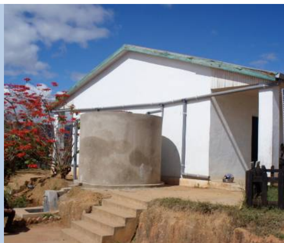
Rainwater harvesting in Madagascar. Gutters lead to a circular storage tank made of plastered concrete blocks. A gravity-fed tap is located below the floor level of the tank.
