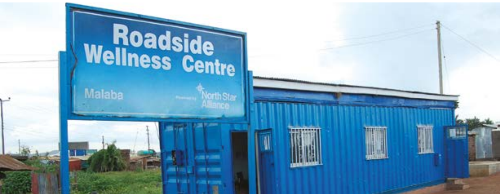
Photo above: USAID supports health services for truck drivers and female sex workers at the NorthStar Alliance Blue Box Center on the Busia border between Kenya and Uganda.
